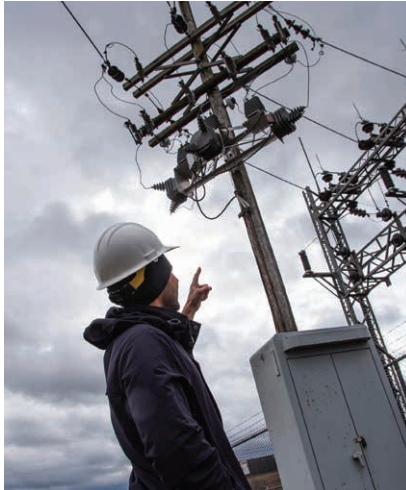
INVESTING IN RELIABILITY: Michael Kovachick, Allegheny Electric Cooperative, Inc. power delivery engineer, examines transmission lines for potential upgrades to improve reliability.
