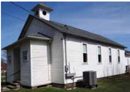
UPDATED BUILDING: The Strongstown Schoolhouse has a new American Standard heat pump unit.
